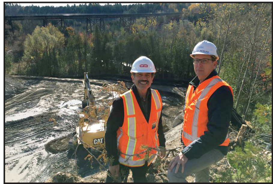
Councillors Butt and Pickles on site of infrastructure construction in Seaton.
